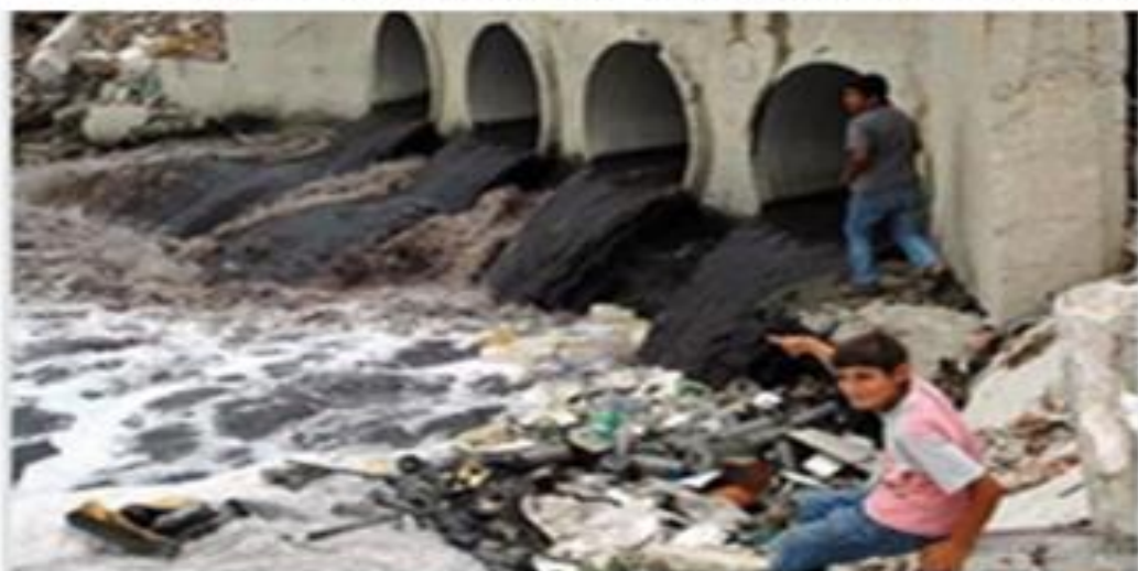
Environmental Awareness; An important approach to prevent environmental pollution.
